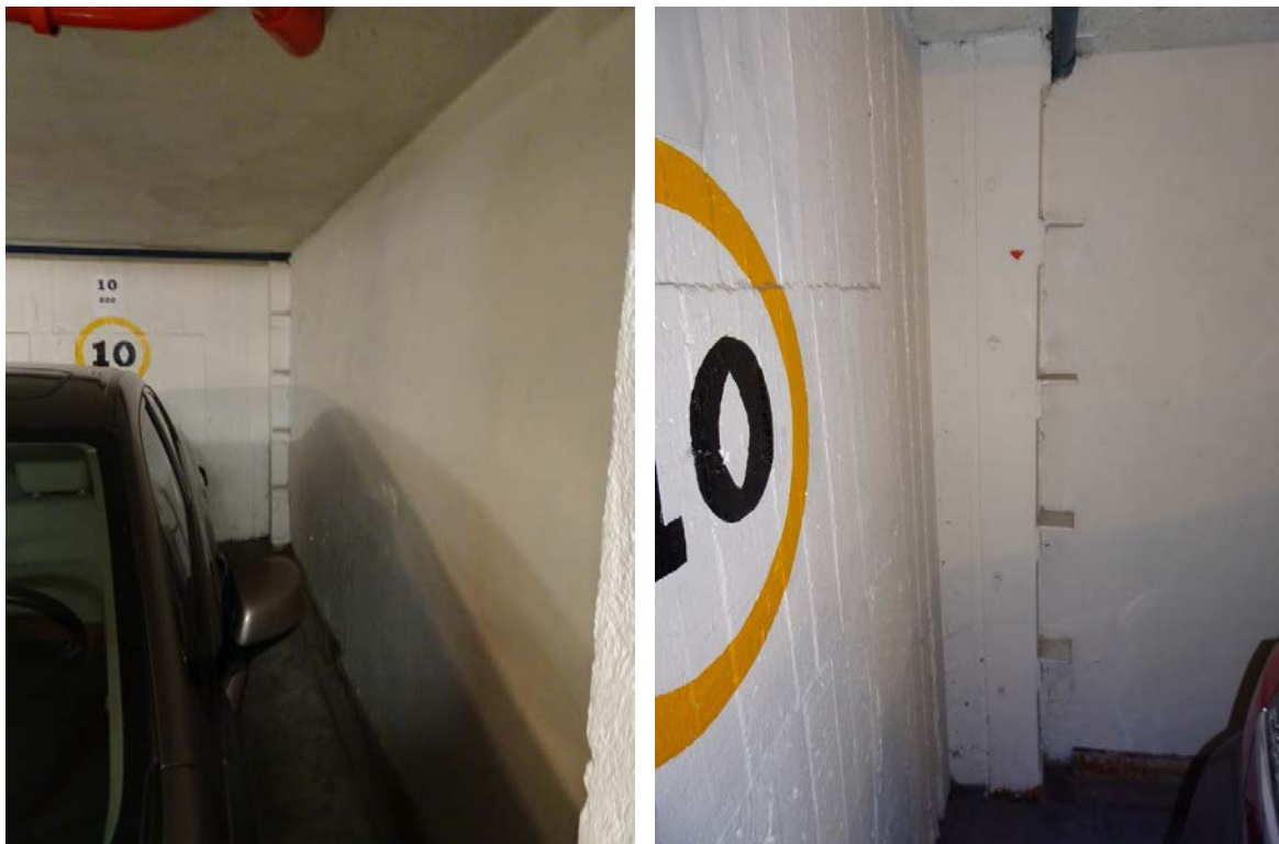
Figure 8: Retrofitted wall in 2017 (left), Steel connection (right)
